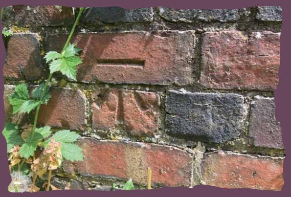
The pre-satellite system has left the nation scattered with surviving 'flush brackets' and 'cut marks' which infilled the network of FBMs. This is a cut mark nearby, on Marsh Drive, on the railway bridge.
